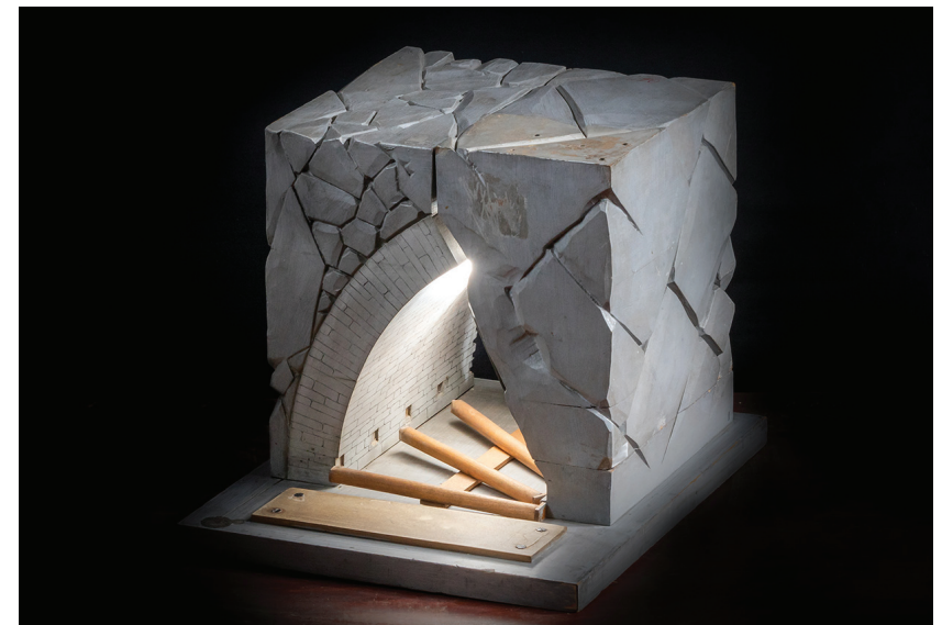
Fig 3. Model of a self-supporting dome. Rubble protection for roadway of soft rocks. Freiberg, Germany, 1820-s. Item belongs to the Mining Museum.
