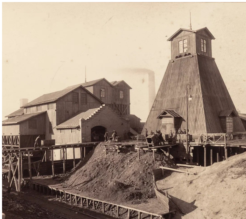
The mine pithead building of the Berestovskaya mine from the side of the access roads. Donbass. Late 19th century. Item belongs to the Mining Museum
