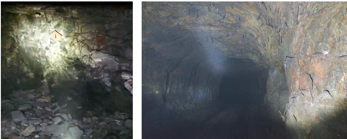
Fig.2. Examples of ore delamination in the border zone under the action of high level stresses
