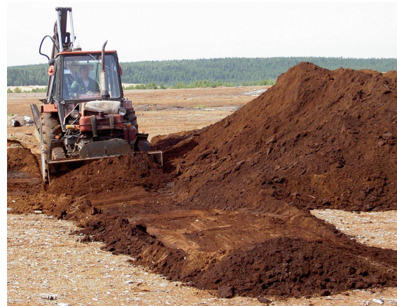
Figure 3. Field testing of lignin excavation and stockpiling
