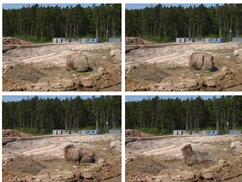
Fig. 6. The sequence of fragmenting boulders with gas generators in the course of constructing an oil terminal
