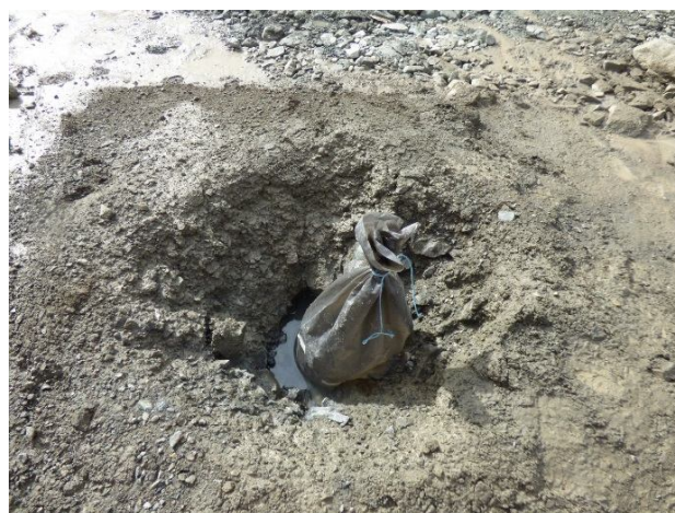
Fig.6. Shell is installed in flooded well and filled with water
