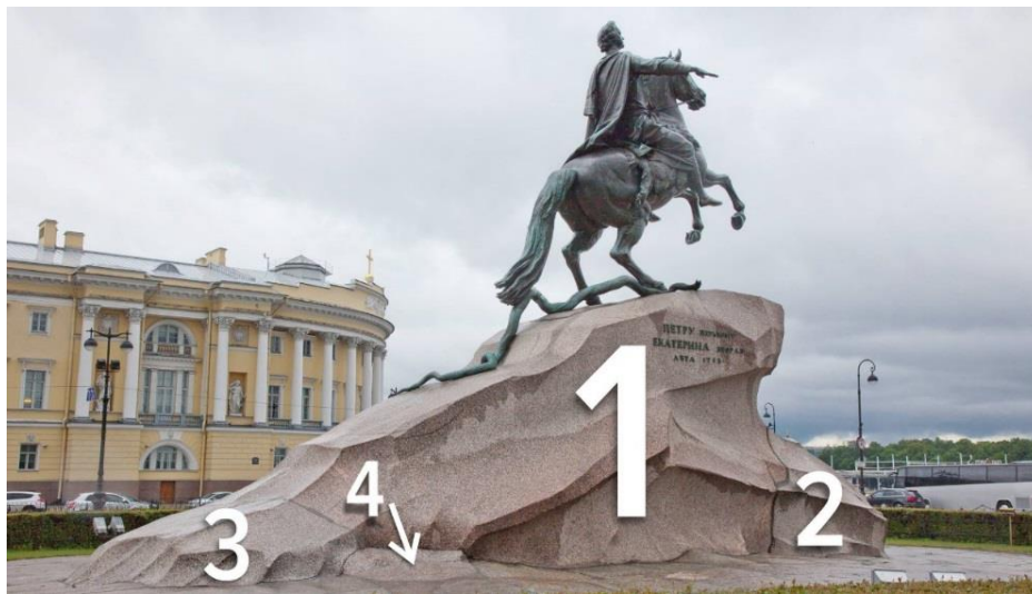
Fig.1. Block structure of the Bronze Horseman pedestal. Photo credit to G.N.Popov, 2016
