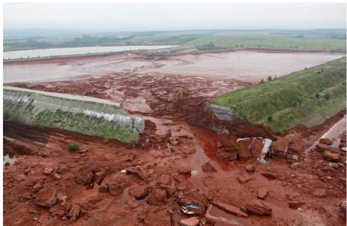
Fig. 1. Ecological disaster: collapse of the bund wall of the red mud storage in Hungary (2010)
